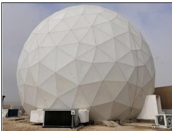
A geodisc radome at Al Udeid Air Base before destruction during the June 2025 Iranian missile attack.
